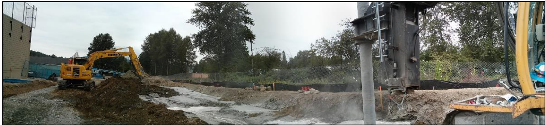
CDSM Installation and Spoil Management
