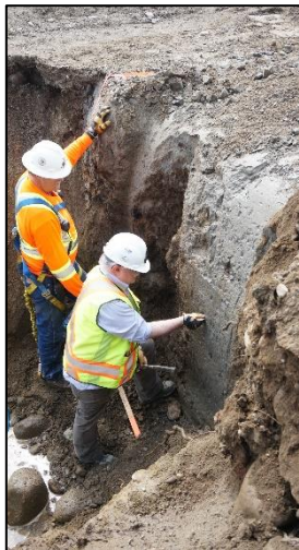
Geotech QA Inspection
