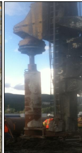
Helical Pile Installation
