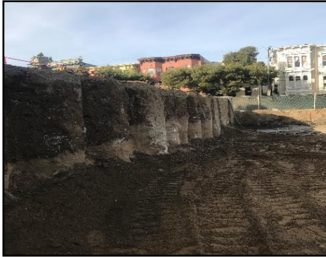
Completed Overlapping CDSM Shoring Wall
