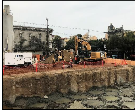
Completed Overlapping CDSM Shoring Wall
