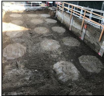
Completed CDSM Elements for Foundation Support
