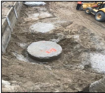
Completed CDSM Elements for Foundation Support
