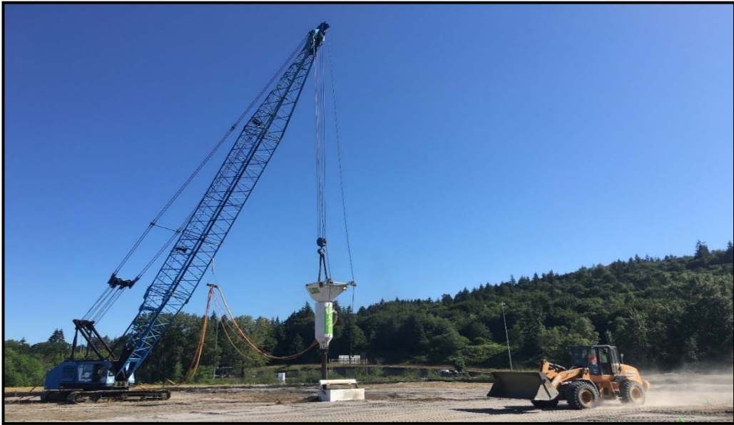
Stone Column Crane and Vibro Probe Installing Ground Improvement Elements
