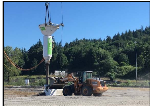
Loader Replenishing Stone Supply
