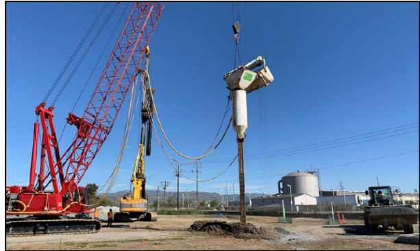
Aggregate Pier Installation
