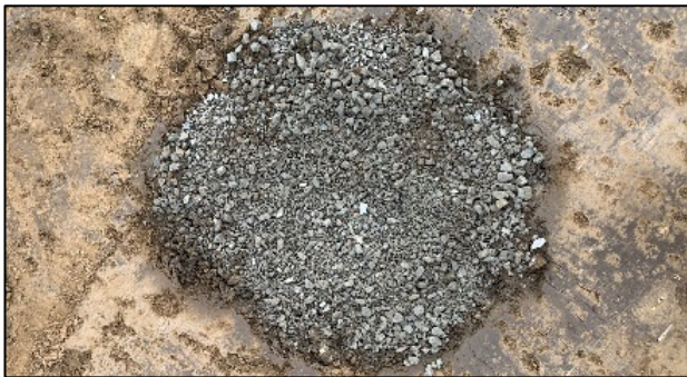
Completed Aggregate Pier
