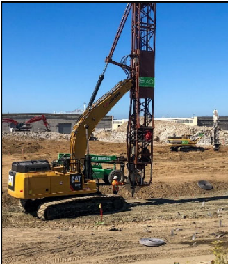
Wick Drain Installation
