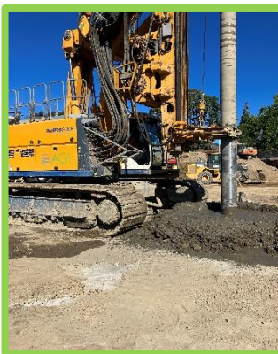
DSM Column Installation
