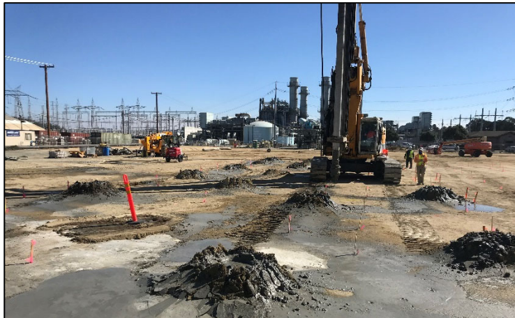
Installation of DGC Elements
