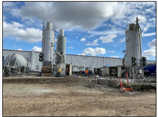
On-site grout batch plant for DSM
